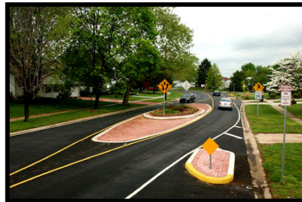
Traffic calming measures can be a simple and effective way to slow traffic
