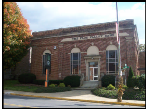
Page Valley Bank Building, 17 W. Main Street – A one-story Classic Revival building constructed in 1928.
